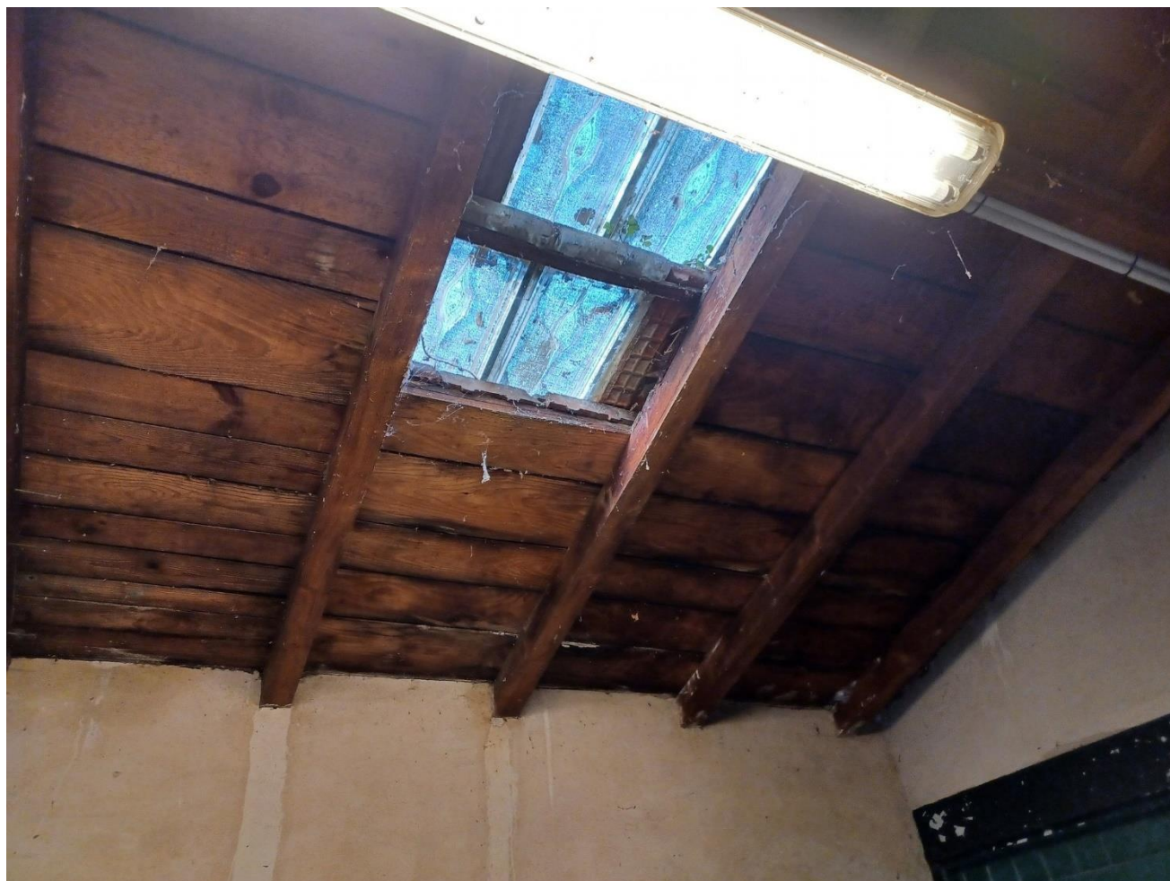
Figure 43: Garage - charpente bois
